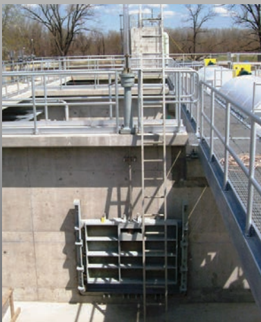
Waste Water Treatment Plant, Missouri, USA 72" x 48" (1.8M x 1.2M) Cast Iron Sluice Gate
