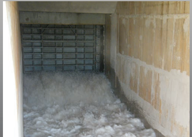
Flow through a partially open 10' x 10' (3M x 3M) Cast Iron Sluice Gate with unseating head
