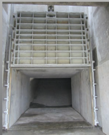
Stormwater Pumping Station, Louisiana, USA 144" x 108" (3.7M x 2.7M) Cast Iron Sluice Gate
