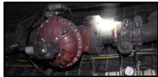
*"Mining and milling present some of the harshest environments for automated valves. Instrument air is not guaranteed to be clean, dry and particle free. Environmental air can be of poor quality and laden with contaminants. Easytork actuators thrive in these conditions and have been used extensively in mining on a multitude of applications."*
