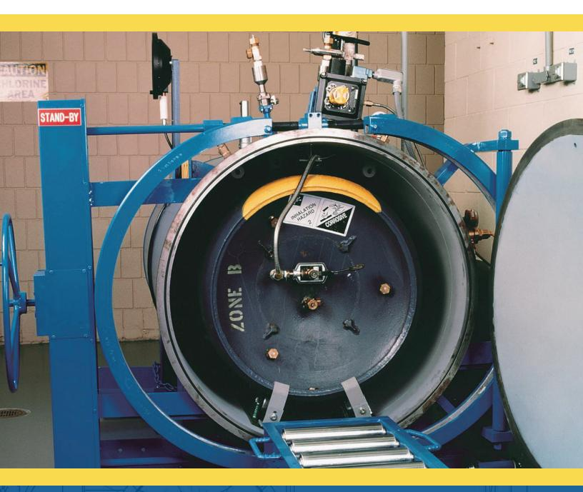
ChlorTainer is a high-pressure containment vessel into which a 1-ton chemical cylinder is processed. If the cylinder should leak, all chemicals are contained within the vessel and processed at a normal rate, so no hazardous waste is generated. Scrubber systems, fans, pumps, tanks, and mechanical systems are not required. ChlorTainer addresses RMP considerations, enhances site security, and provides fail-safe protection for plant operators.
