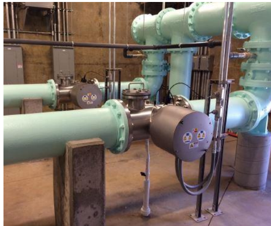
Medium pressure with lamps perpendicular to flow
